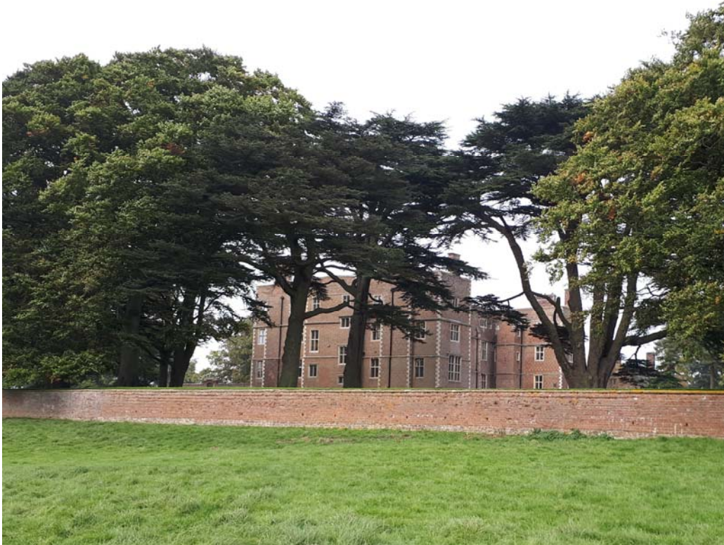
Photo 5: A view of the Ha-ha wall and the Hall from the bridleway which at this point is around 30 metres away from the wall.
